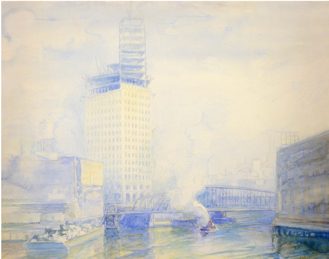
Charles Biesel (American, 1865 - 1945) View of Wrigley Building Under Construction From State Street Bridge, ca. 1920 Watercolor on paper 15 1/2 x 19 1/2 inches #7674
